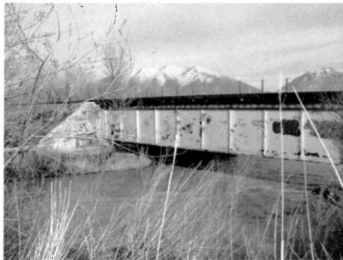
Deck Girder (Less Water Flow)
