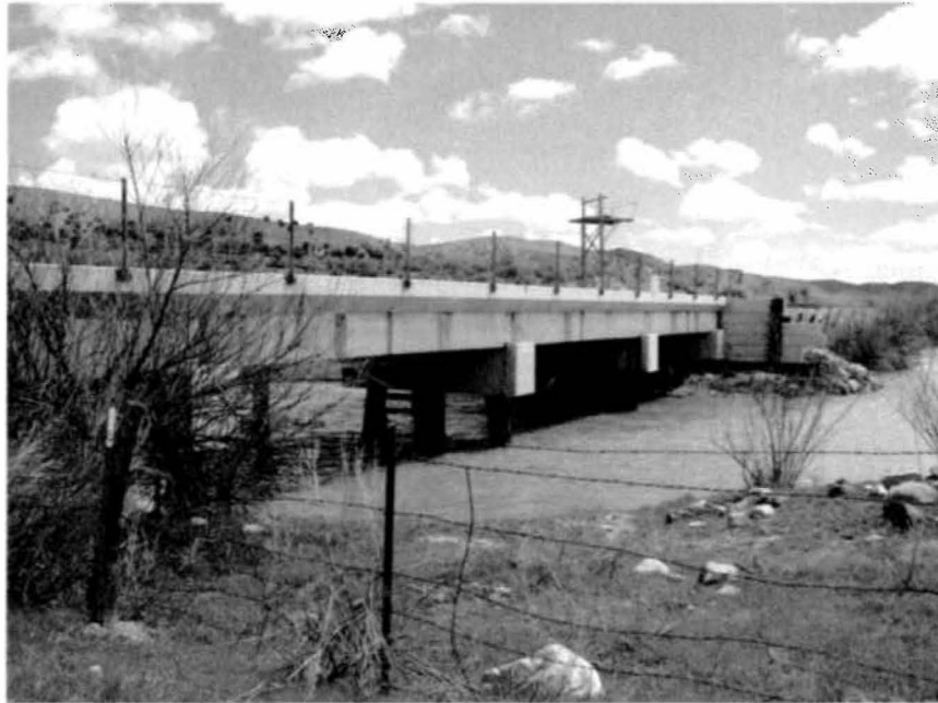
Precast Concrete (Greater Clearance and More Water Flow, even with an Additional Pier)
