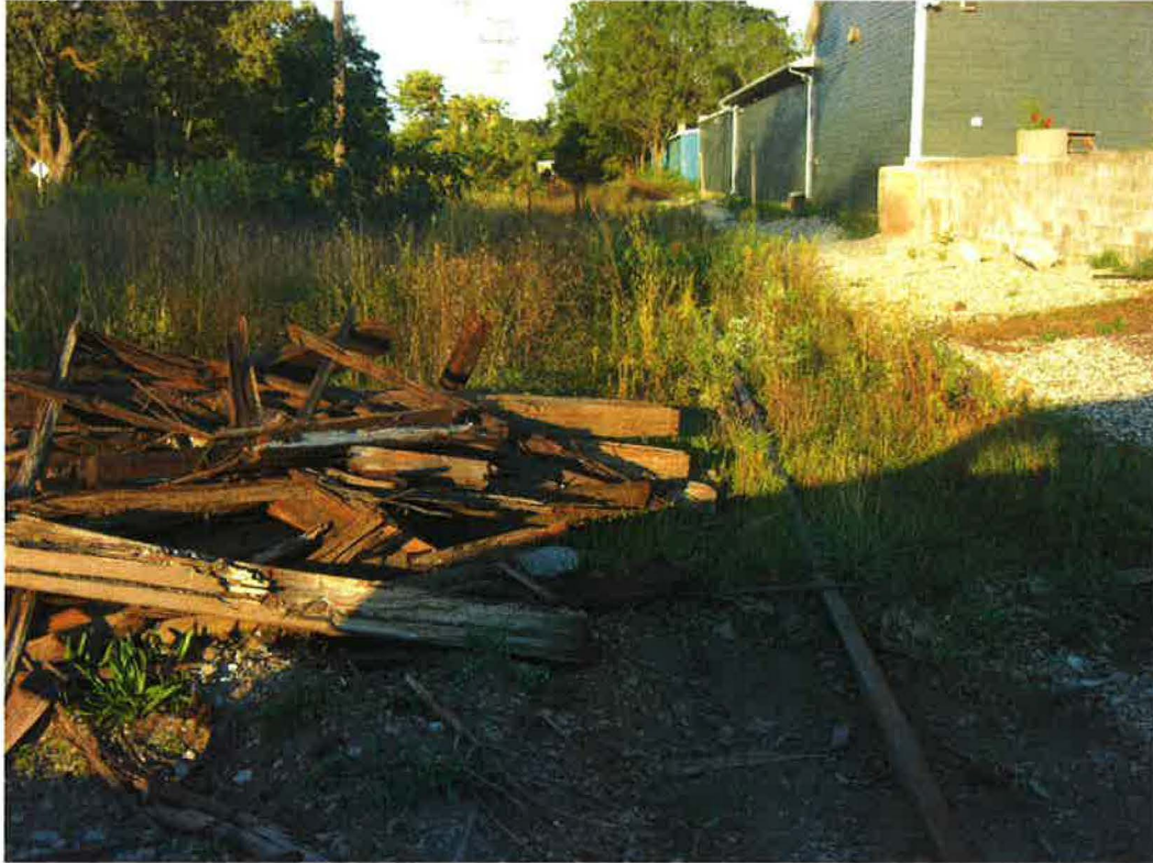
Figure 6-10. Abandoned rail line to the Option R3 site.
