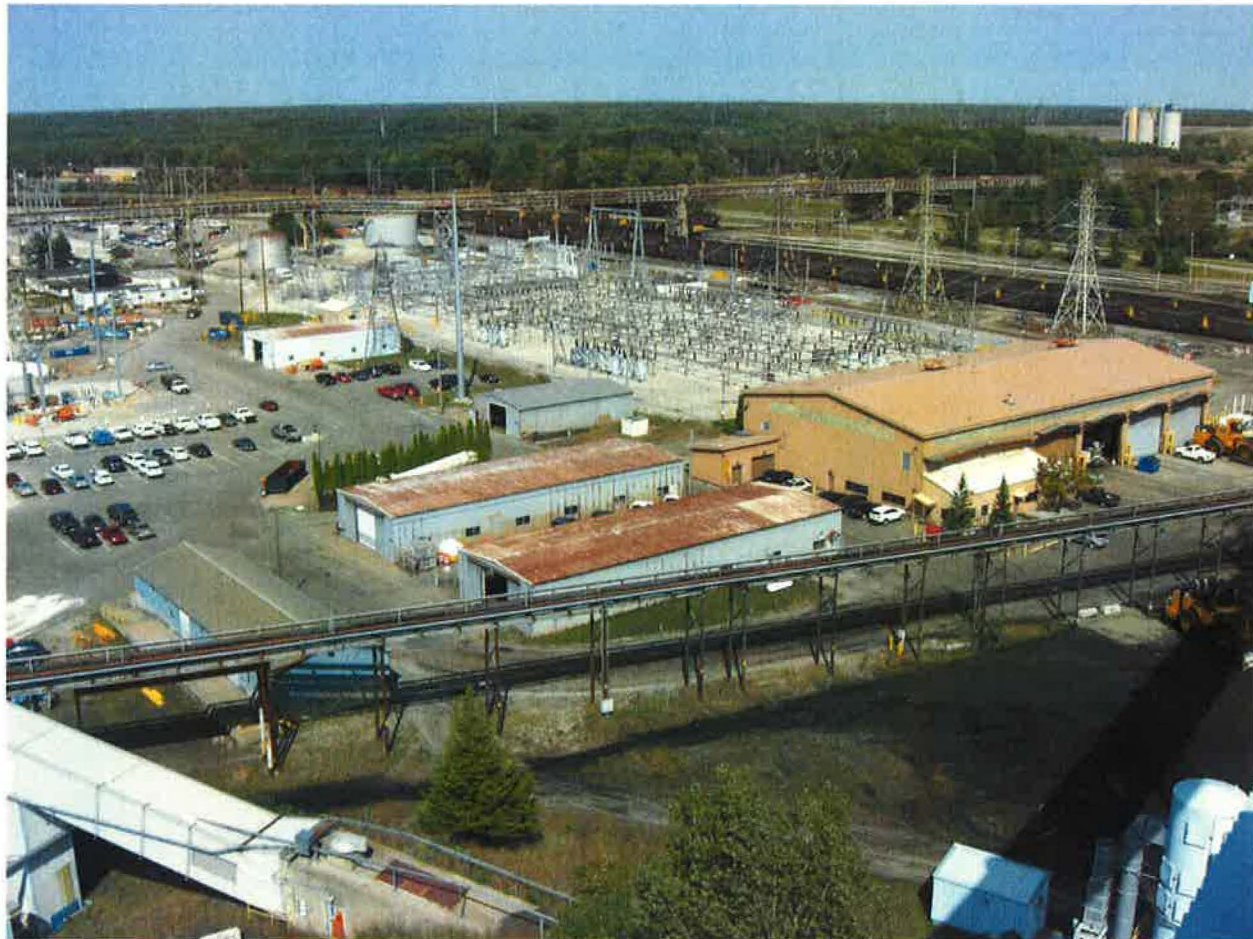
Figure 3-14. Area north of existing stockpile would require relocating switch yard and other facilities.
