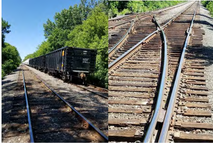
Looking west, Stored pellets and empty gons
