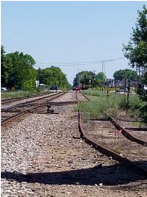
Salt Track turnout
