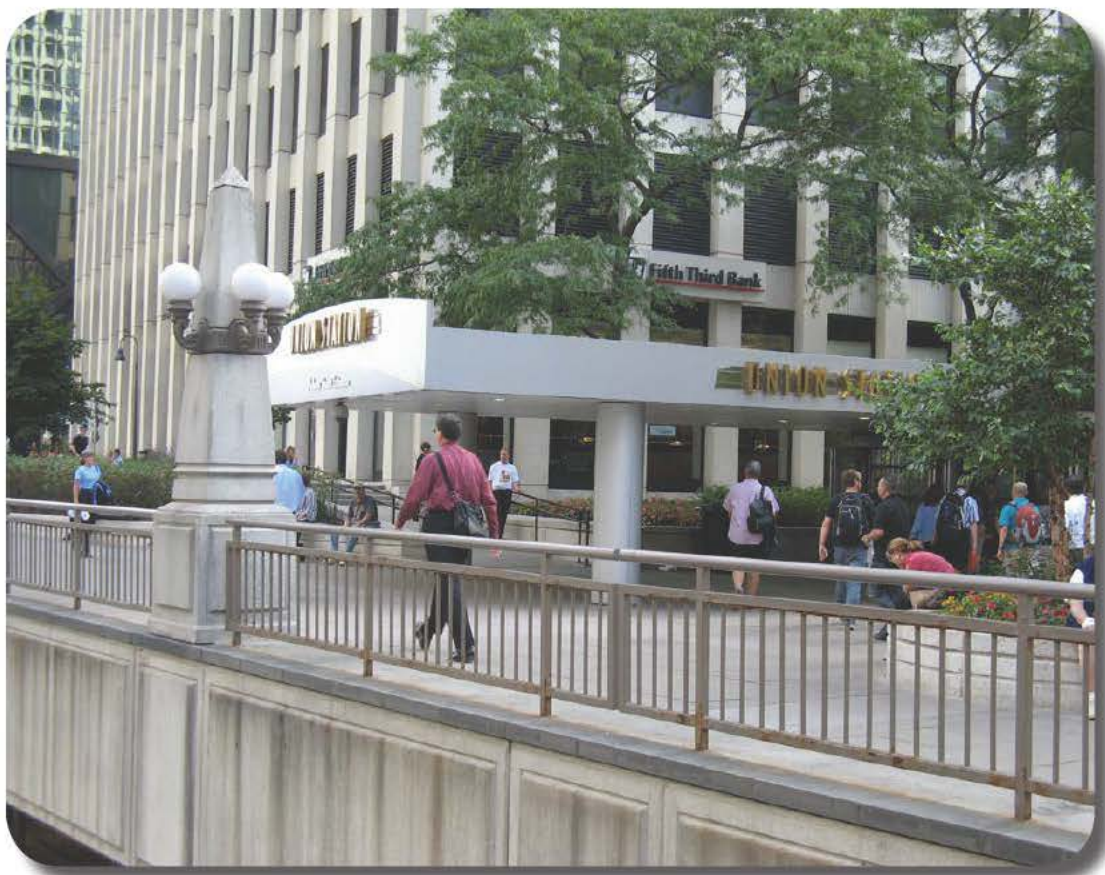
Entrance to Union Station near W. Adams Street, existing conditions
