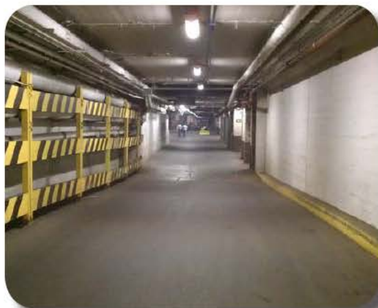
Existing below-grade passageway could be upgraded for passengers using converted mail platforms
